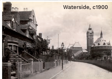
The Old Ferry House
